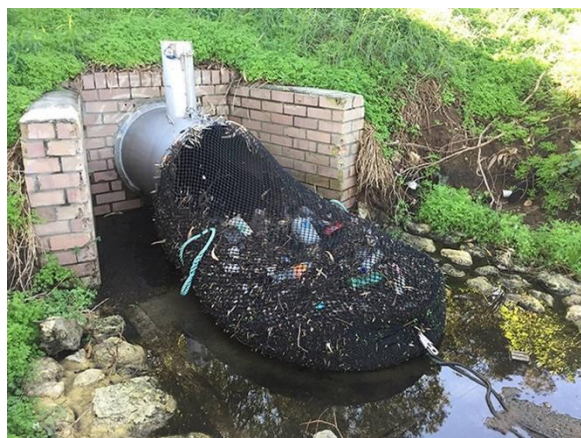
Figure 4. Drainage nets, Australia
